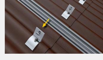
2. Mounting the vertical universal profile (UP-X) The pre-assembled universal profiles are then securely screwed onto the TS-COR using the M10 hammerhead screw.
