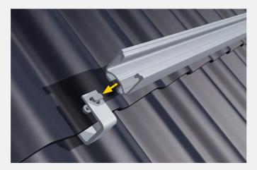
2. Mounting the vertical base profile (UP-L) The pre-assembled profiles are then securely installed on the roof hooks with the M10 hammerhead screw.
