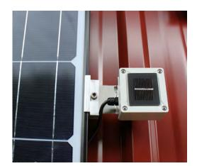
Spektron 210 is fastened with the bracket on the mounting rack of the PV system. Care must be taken that the sensor has the same inclination and orientation as the PV system to be examined. Minor deviations may result in measuring errors!
