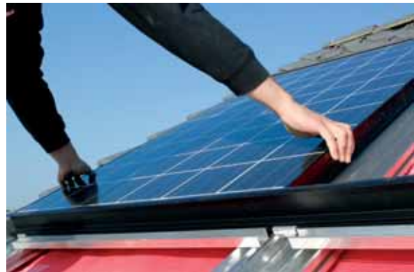
Simple insertion of the modules
