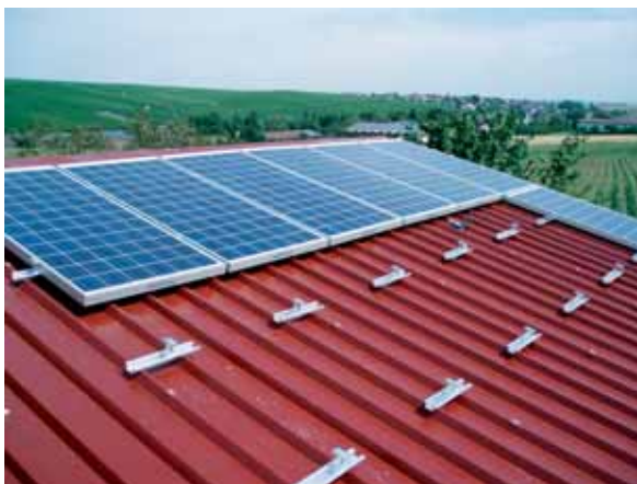
The TRI-VENT support profiles are only riveted to the roof at the points required by the module installation.
