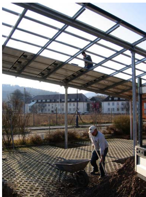
Construction of the SolarCarport began in February 2007.
